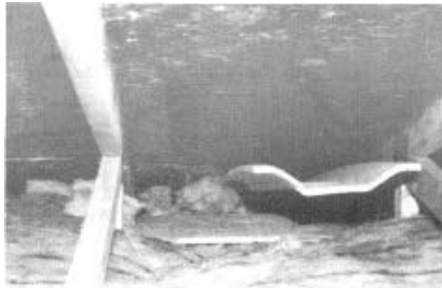
Saturated roof sheathing blackened by mold and beginning to sag.
