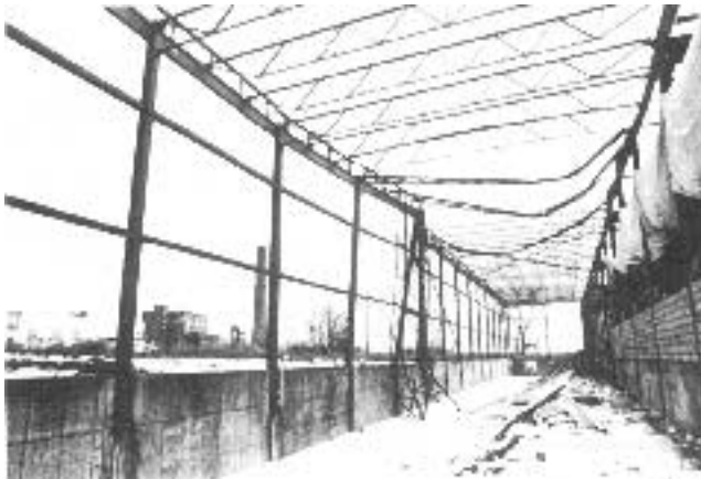
Twisted joists on the job site: a lousy way to start the week.
