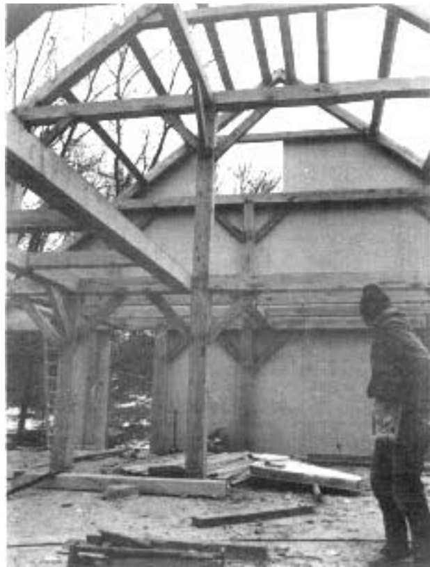
Ancient art joins modern technology in many timber-frame homes, such as this one, which combines hand-worked oak timbers with urethane-core stress-skin panels. The house was built by panel maker Bud Couto of Atlas Industries in Lunenburg, Mass.
