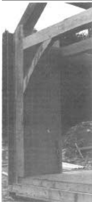
A hefty oak post, end girt and knee brace mortised and tenoned and pegged for a rugged and attractive joint.
