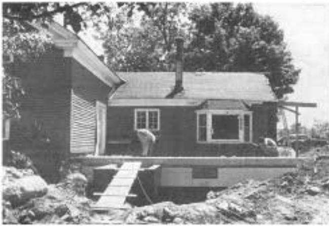
Workers finish up the floor deck of the new 10x24-foot addition.
