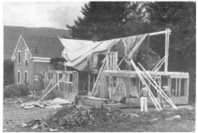
Plastic tarps draped over a temporary ridge kept the building dry through the long delays caused by plan changes.
