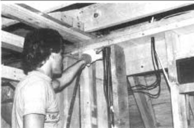
A PEP employee seals a potential "attic bypass" where a plumbing stack penetrates the top plate in a new home.
