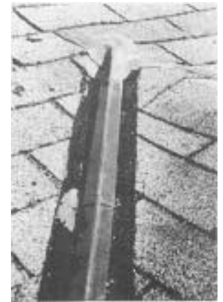
The completed job, with lead flashing at the joint of the two valleys and the U-shaped valley cap in place. The old, tar-coated valley is still visible.
