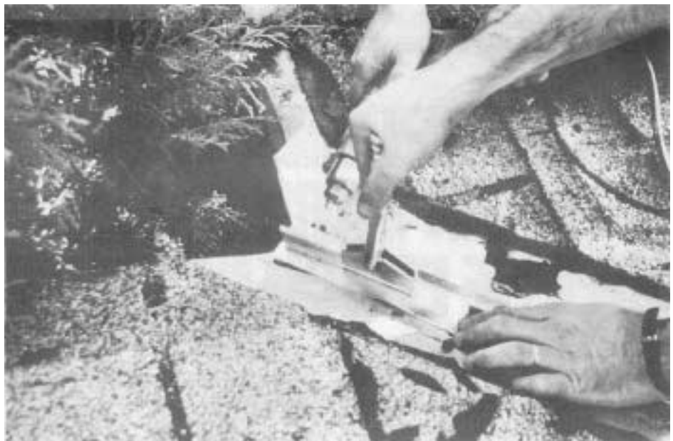
With the new inverted-U cap in place, a carpenter squeezes the pieces shut while another worker drills a hole for a pop rivet.
