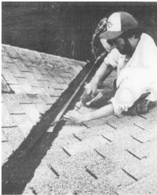
A carpenter inserts replacement pieces on one side of the old valley.
