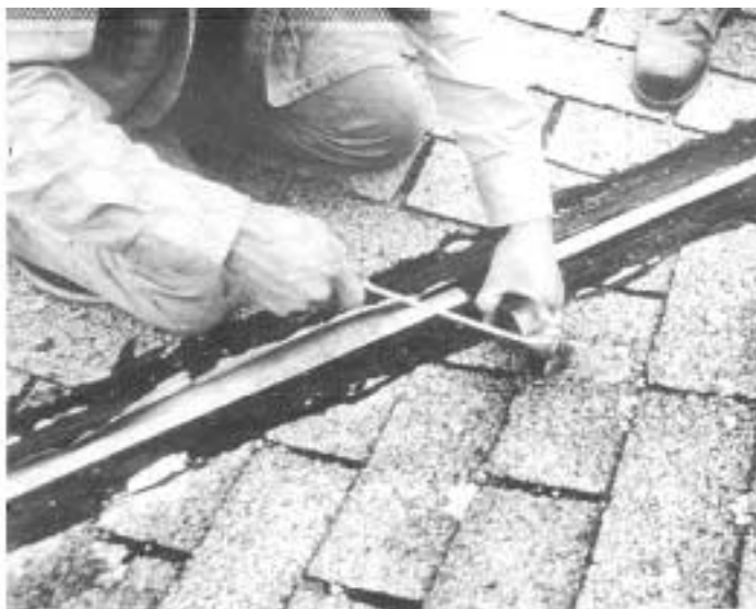
Phase 1 of a new valley-repair technique. At left, the old valley is cut with a masonry knife. Above, with the old valley cut, a new piece of flashing is inserted on one side.
