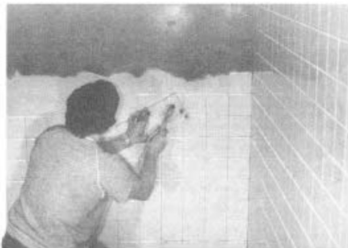
To ensure good contact between tile and thin-set mortar, a tradesman sets each tile with a hard rubber mallet and a "beating block."
