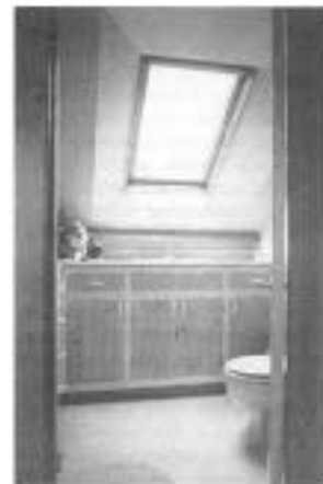
The splayed opening effectively reduces glare and lights a wider area.
