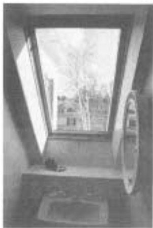
This skylight creates headroom over a sink in a tight space.
