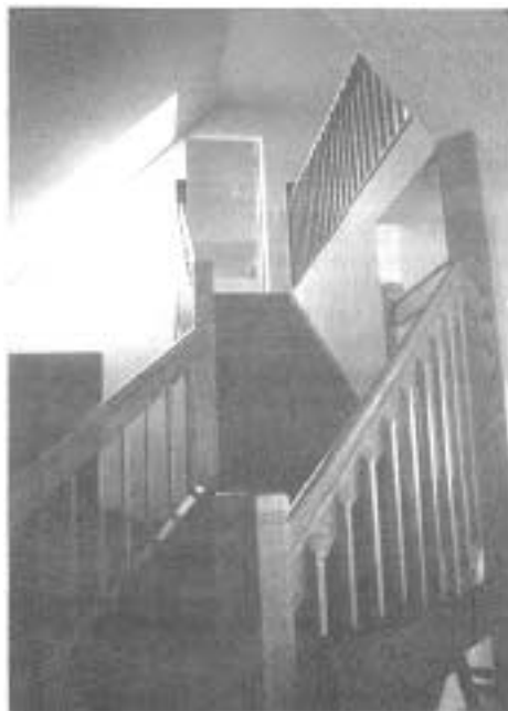
Stairwells make convenient light shafts for bringing sunlight into interior rooms. Placing the skylight next to the wall makes an effective reflector and reduces glare.
