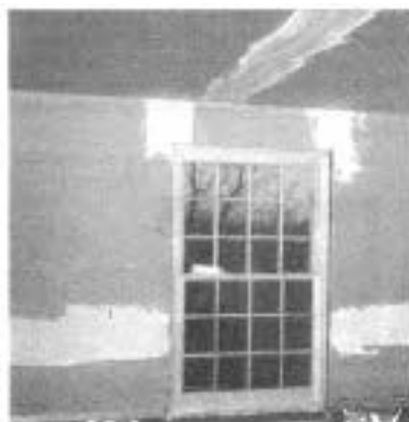
The first step, after hanging the board, is to put a thin coat over all the joints except corners.
