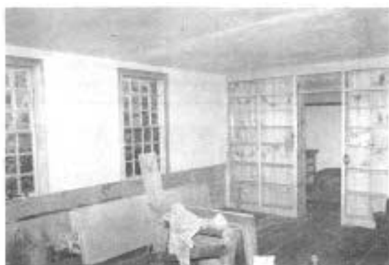
Next, the walls and ceiling are coated with about 1/8 of an inch of plaster. The author prefers to install the moldings first and finish the plaster to the wood.
