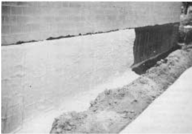
Enkadrain subsurface drainage mat prior to backfilling.
