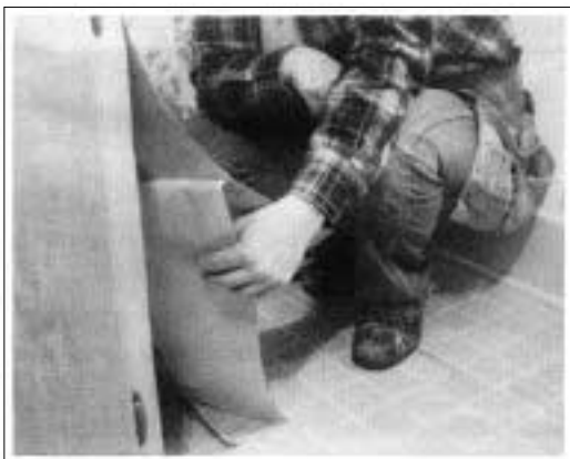
↑ Step 3. After checking for fit, the peel-off backing is removed and the veneer stuck in place.
