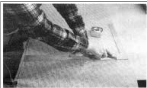
↑ Step 2. After measuring the cabinets, we cut the pre-finished oak veneer, big pieces first.
