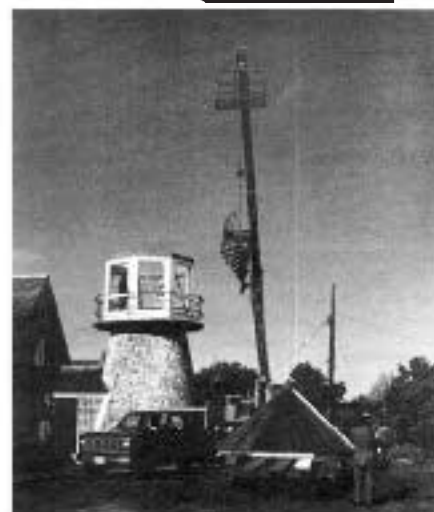
4. Meanwhile, sculptor Piper had fabricated a spiral stair—designed to drop through the freshly sawn hole atop the lighthouse—with just a couple of inches tolerance.
