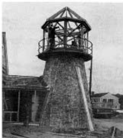
3. The roof was framed in place for an accurate fit, then removed to receive its standing-seam copper finish. An ornamental copper globe with a spire was added later to cap off the roof.
