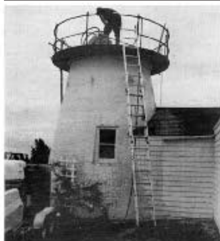
1. The first job was to cut through a couple of feet of concrete at the top of the 17-foot tower to create a larger stair opening. The original masonry stairs terminated halfway up and ended with a ladder.
