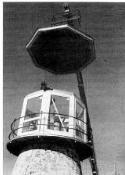
5. After lowering the stair, the copper cap is gingerly set in place—raising the height of the tower to 30 feet.
