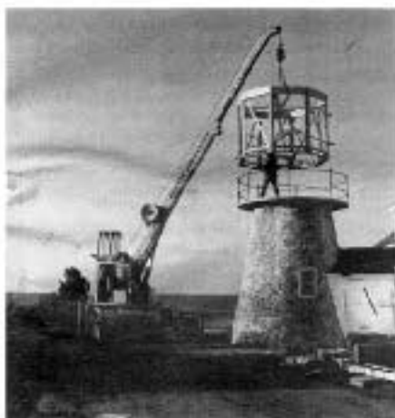
2. The octagonal frame was assembled on the ground and lifted into place—with openings for eight 4x6-foot windows. (Every other window has an operable awning panel at the bottom for ventilation. One window is split into two sets of double casements for emergency exit.)
