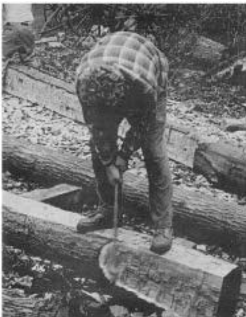
Only butt logs from oak trees are suitable for gunstock posts. Here a restoration worker scores the log with a scoring ax—the first step in the hewing process.
