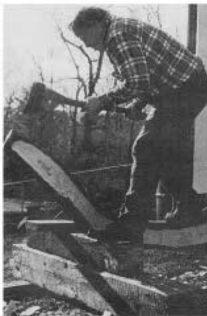
From apple tree to signature brace. Master barn builder Richard Babcock smooths a scored log with a hewing ax (above,) and finesses the final finish (right) with an adze
