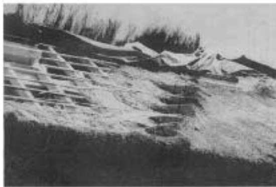
A thatched roof is built up in courses. In this case, bunches of water reeds are held in place by split hazel "sways," which in turn are hooked to the open rafters and covered by subsequent courses.
