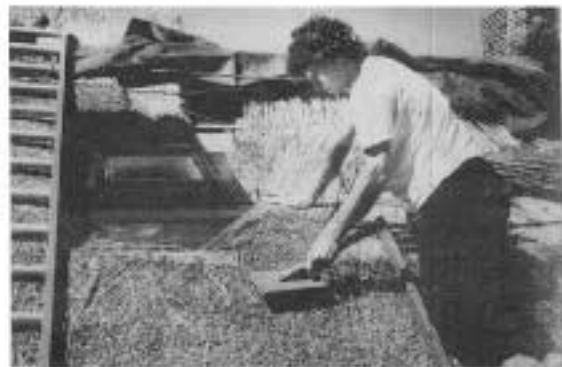
A thatched roof is built up in courses. In this case, bunches of water reeds are held in place by split hazel "sways," which in turn are hooked to the open rafters and covered by subsequent courses.
