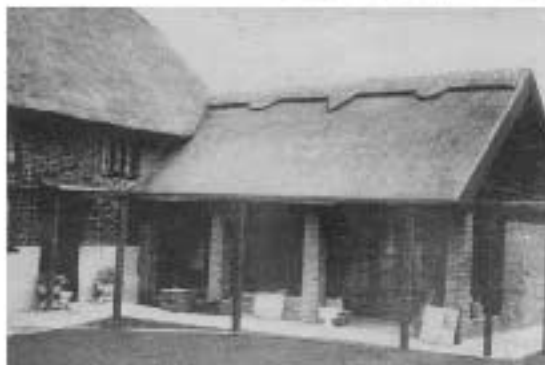
B ecause of its steep pitch, the roof on the left is thatched with long straw. The new addition employs water reed. Note the thatcher's trademark, the elaborately decorated cap.
