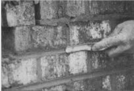
Concave or V-notched joints help the joints resist moisture and look good.
