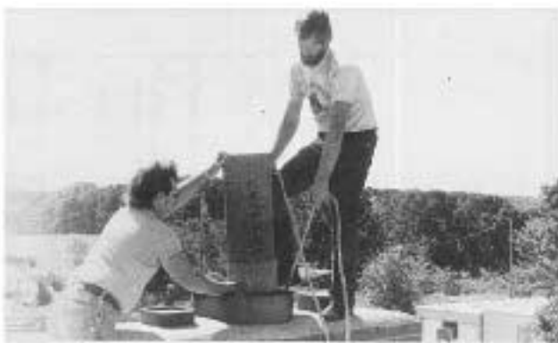
Two-foot sections of the Chintek liner (an American-made clone of the Iso-Kaern liner) are connected with metal collars and lowered down the chimney. The flue tile uses volcanic-pumice aggregate, and is insulated with a mixture of clay pellets and cement.
