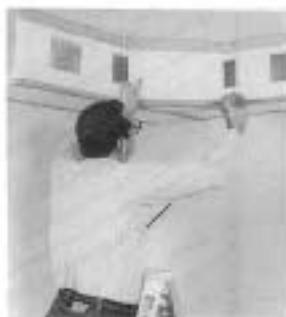
**Polystyrene soffits** promise easy installation and low unit costs. Builders can buy Ultra-Soffit at \$3 a linear foot. According to its manufacturer, 8 feet of soffit can be installed in 15 to 20 minutes with just 24 screws. The soffit can be cut or trimmed with ordinary tools, and is adaptable to both standard and custom cabinet depths. Corner soffit pieces are also available. For more information contact Epsco, 4080 First Avenue, N.E. Suite 105H, Cedar Rapids, IA 52402; 319/364-2000.
