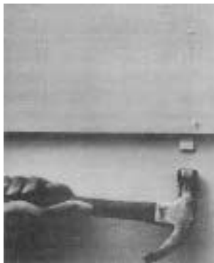
When insulation is blown into existing wall cavities, paint problems can be avoided by driving plastic wedges between the siding laps at each stud. The separation promotes drainage and drying, and prevents capillary suction of water into the lap area.
