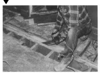
Temporary jacks downstairs hold the sagging beam true while the epoxy cures to permanently hold it in place. Interruption to the existing ceiling was minimal.
