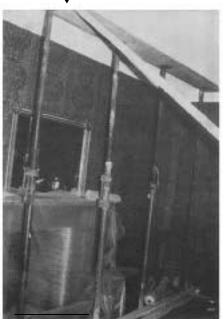
Repair in-place with steel and epoxy is sometimes the best treatment for decayed wooden beams.
