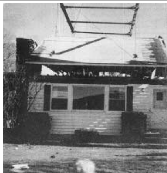
Using a custom lifting frame, house mover Royce Lanphear picked up the first half of the roof with four cables tied around lengths of 6x6 braced in place near the eaves. The 20-foot section was stored on the ground while the pre-framed walls were raised
