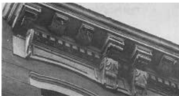
The missing consoles and brackets had surfaces that trapped water, dooming them to failure. What's left are sparrow motels.
