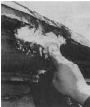
Epoxy filler, properly applied, can reproduce proper cornice contours.
