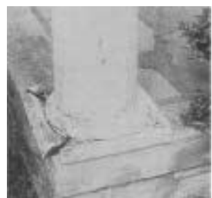
The bases of wood columns should be detailed to sit off the deck. Otherwise, water is wicked into the end grain.
