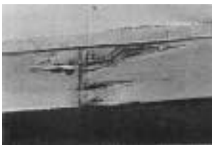
All exterior millwork should be coated with a WRP before painting. End grain—the most vulnerable part—should be dipped.
