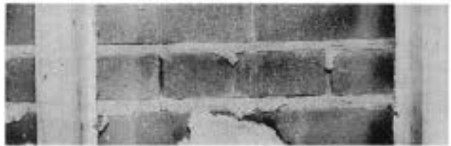
Fig. 3. Sandblasting removes smoke residue and char in cavity between wall
