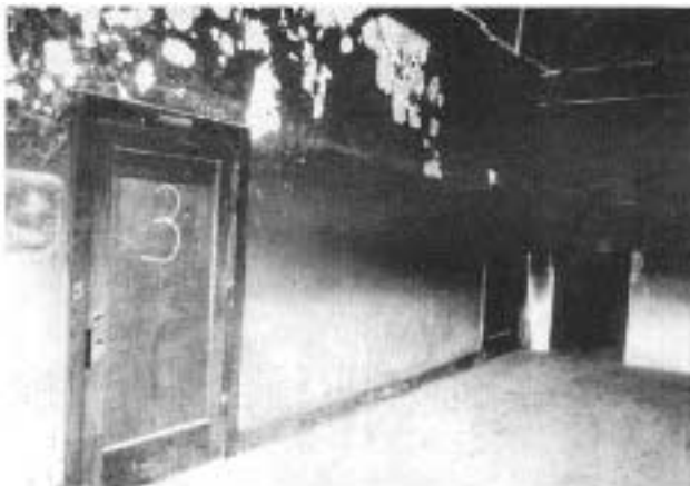
Fig. 4. The central hallway of the McGuffey Art Center in Charlottesville, Virginia was badly damaged during a fire.
