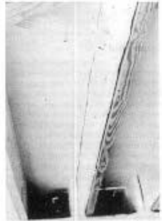
Fig. 2. Sandblasting charred lumber and laminating new structural member to old is a cost-effective alternative to replacement of ceiling joists.
