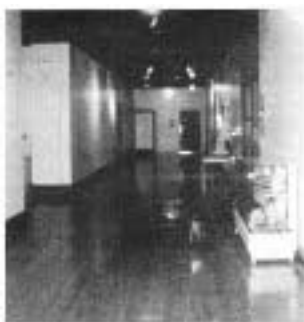
Fig. 5. Sandblasting removed damaged portion of walls. Bonding compound was applied, followed by new coat of plaster and resinous sealer.
