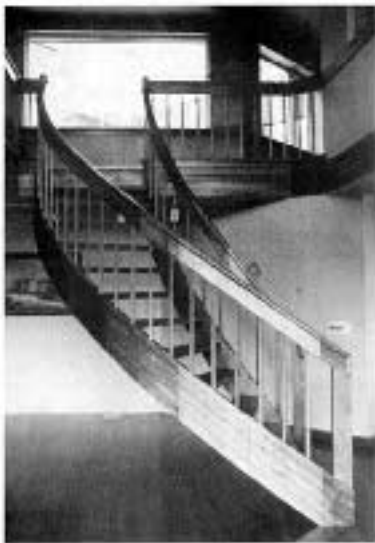
The finished circular stairway turns 90 degrees. The radius of the outer stringer is 89 inches.
