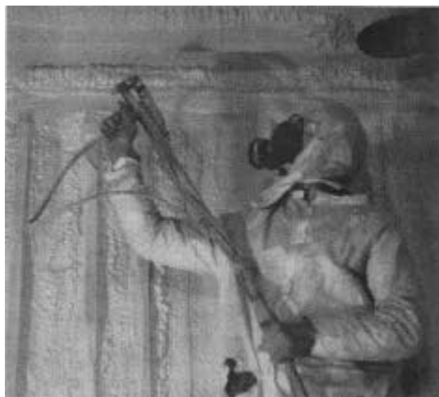
Urethane insulation is sprayed on in thin layers called "lifts" that build up to the desired thickness.
