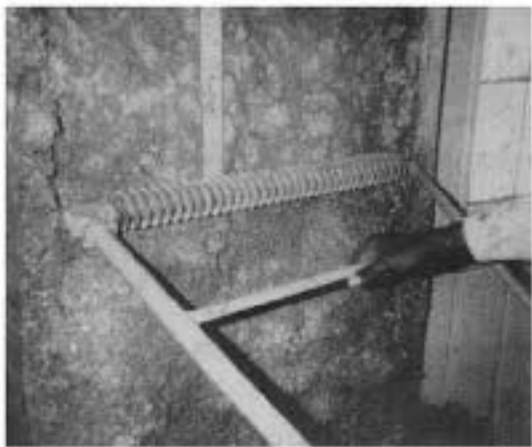
After spraying the cavities, the excess cellulose is mechanically removed with a "scrubber," (above left) and fed back into the hopper. The result is a clean wall (above right) ready for vapor barrier and finish.
