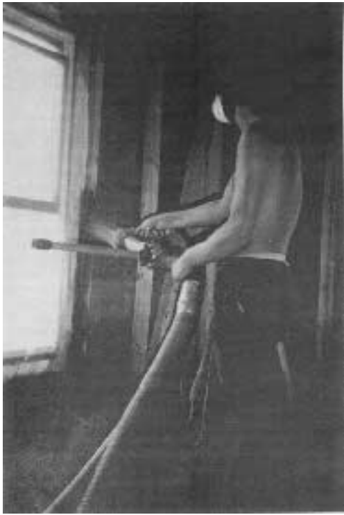
Spray cellulose fills stud cavities completely, sealing off most air leaks and preventing convection within the wall.
