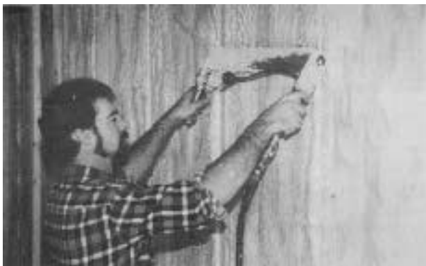
Excess urethane insulation can be planed with a pneumatic device.
