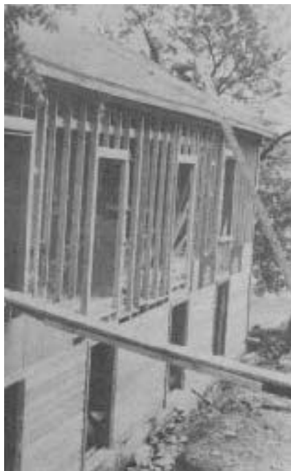
View of the east wall being reconstructed with the balloon framing.
