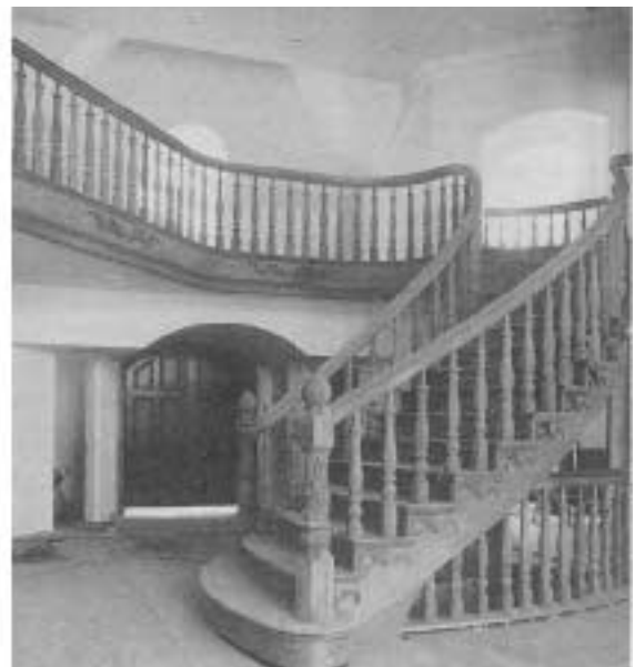
The wood carvings featured on many Woodsmiths stairways are roughed out with power tool and then finished by hand.
