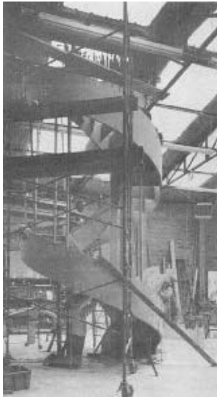
Workers at the Woodsmiths plant assemble a three-story-high stairway as a single unit. Taller structures are built in separate sections.
