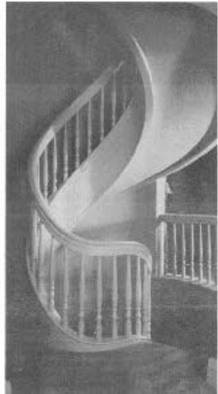
Stairways with complex curves are often plastered underneath although Smith says that wooden soffits can be built for any stair if the customer prefers.
