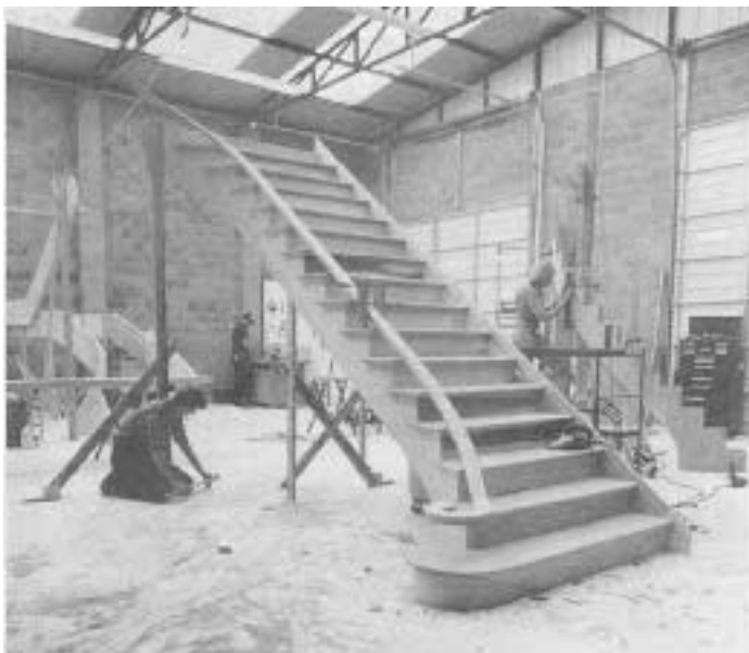
The railing—complete with volute—is carefully fitted to the stairs before balusters are installed. Despite its elegant details, this is one of Smith’s least expensive stairways.
