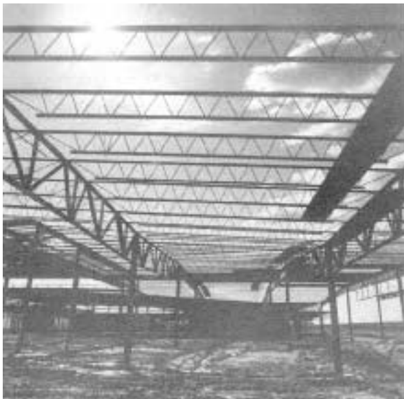
Bar joists can span up to 50 feet on 8 foot centers in most parts of New England.
