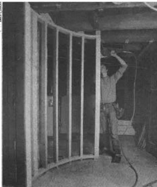
The author used plywood top and bottom plates for this non-load-bearing curved wall.
