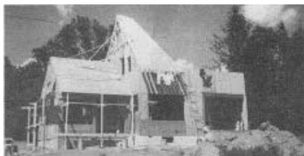
Preassembled rafter pairs lean on the gable-end wall and await final positioning. After they were set in place, the kneewall bowed out 1/2 inch in the center and might have kept going without the aid of a come-along and a strategically placed brace.
