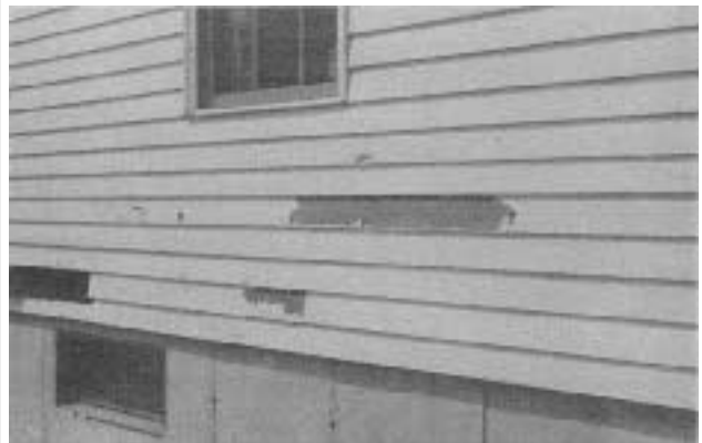
Completed in the fall, this Mass. house started peeling badly by mid-winter. Two problems are cited: high interior moisture levels, which caused peeling, and incompatibility of primer and paint (actually white stain), which caused the two to separate. Each paint company blamed the moist wood—and the other paint product.
