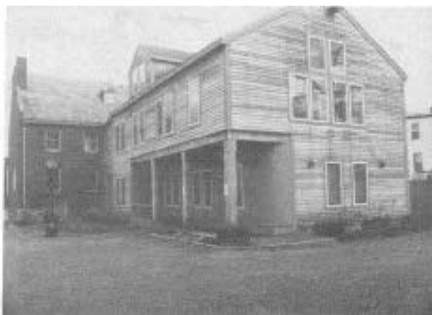
Construction took five months. To comply with the wishes of the Division of Historic Preservation, the addition had to be reduced in height, made aesthetically compatible with the original house, and be mostly out of view from the street.
