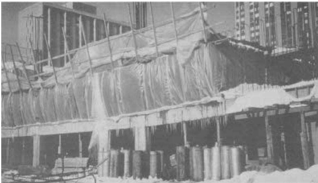
In cold weather, buildings should be enclosed while concrete is placed and cured. Canvas tarps are rugged, but translucent polyethylene sheets are sufficiently strong and will admit daylight.
