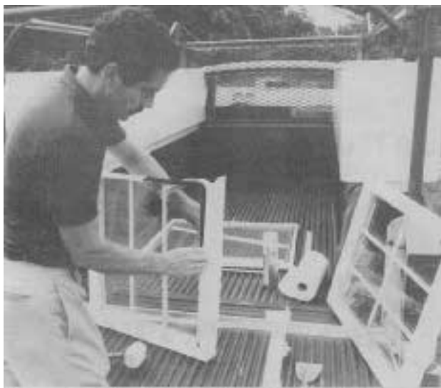
The author can replace a fogged glass unit on their vinyl replacement windows in about 10 minutes.
