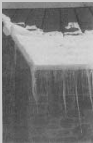
If you like metal roofing, use standing-seam — not corrugated or V-crimp — which are prone to condensation underneath. But metal roofing, along, will not cure ice dams.
