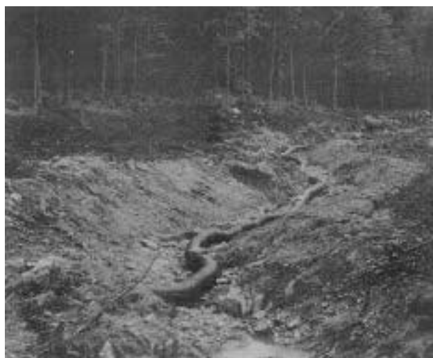
In this ski area, a stream is being temporarily diverted through corrugated ADS pipe, while a new stone-lined channel is being constructed elsewhere on the site. This inexpensive pipe can also be wed to divert spring runoff around an exposed building site.
