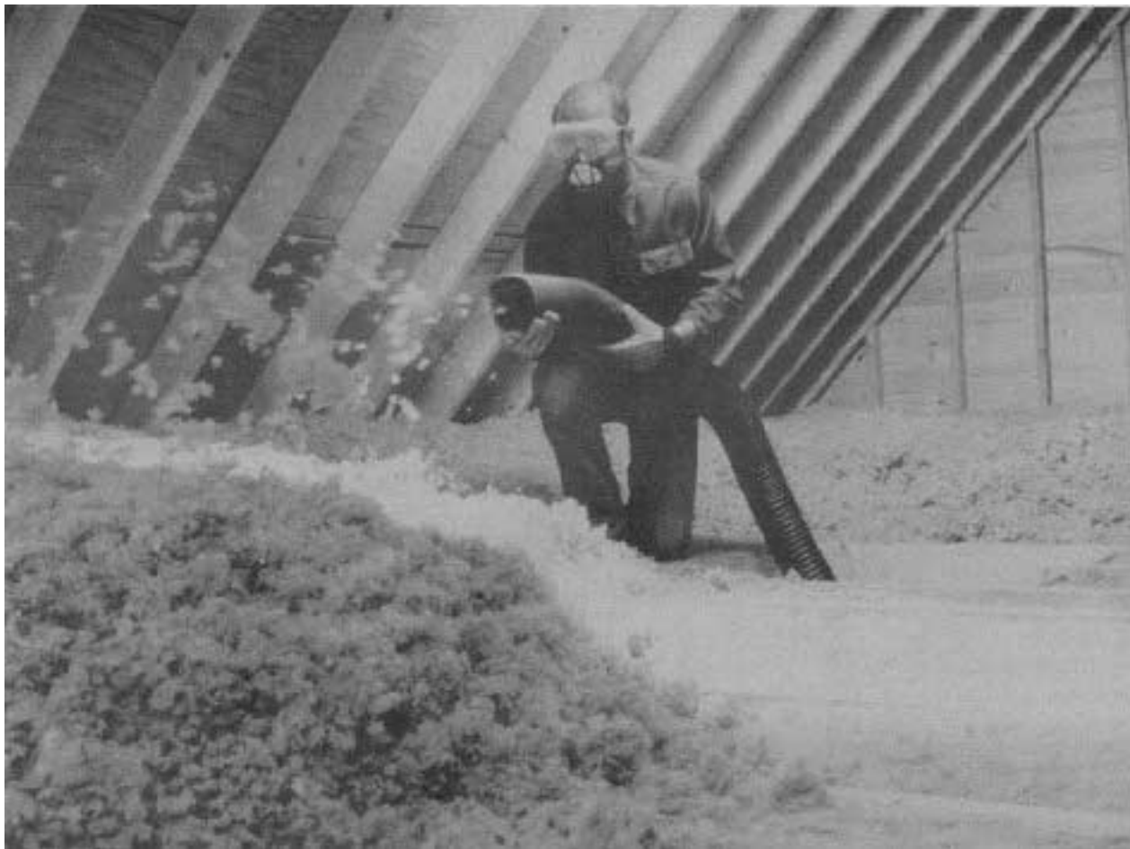
Installers of blowing wool—mineral wool in particular—might face health risks. But batt installers are probably safe from harm.
