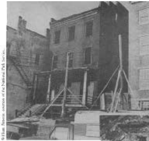
The James Breed House, a circa 1848 rowhouse located in Norwich, Connecticut, suffered a major fire in early 1985 which severely damaged the interior, including the main stairs (inset).
