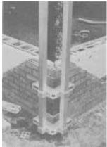
Assemble brick and block corners faster with this self-supporting 10-foot-high corner system. The entire assembly can be moved as a unit to any height required. According to the manufacturer no nails or braces are needed, only a level to plumb the 10-foot poles. The product promises to provide up to 40 percent savings in labor costs. For info, contact Goldblatt Tool Co., P.O. Box 2334, Kansas City, KS 66110; 913/621-3010.
