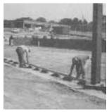
Designed to become integral with the floor, Permaban concrete screed rails are left in-place when pouring the floor. The concrete used in constructing the rails is stronger than the surrounding slab and provides a 40-percent greater load transfer and reduced joint spalling. The rails can be used in any slabs on grade, on metal decks, and in slab construction where tilt-up walls are installed. For information, contact Permaban North America, P.O. Box 1411, Matthews, NC 28106; 704/821-7000.
