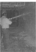
Designed to end wall voids and provide sound insulation this product is spray-applied. ThermoForm is a cellulosic insulation treated for fire retardancy that contains its own adhesive. Once applied, the insulation is "scrubbed" level with the studs. Based on ASTM testing 2.5 inches of the product has an R-value
