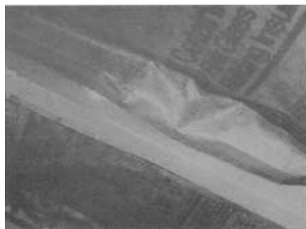
Figure 6. If paper faced batts are pushed up too tightly against the roof, the airflow through any notches will be blocked. To keep them open, you can box in the notches with hardware cloth (see Figure 3)
