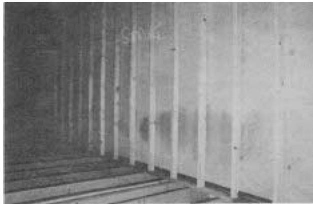
Figure 1. Furring of basement walls and stuffing with fiberglass is easier than exterior insulation—and performs about as well.
