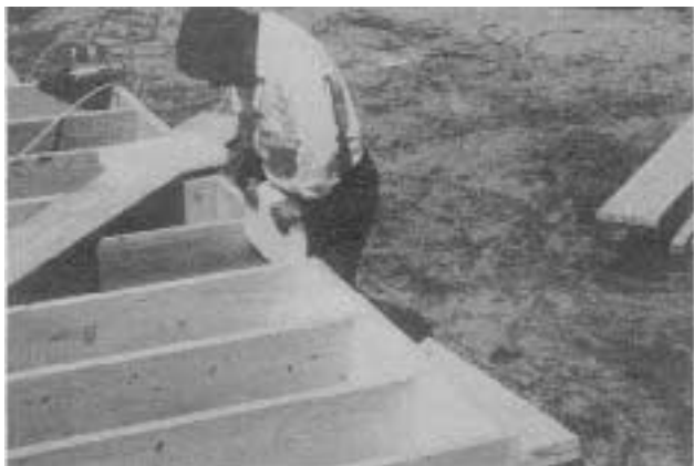
Figure 2. Compressible foam Sill Band Sealer is most efficiently installed from the top during the framing. Unfaced fiberglass is added on the interior.
