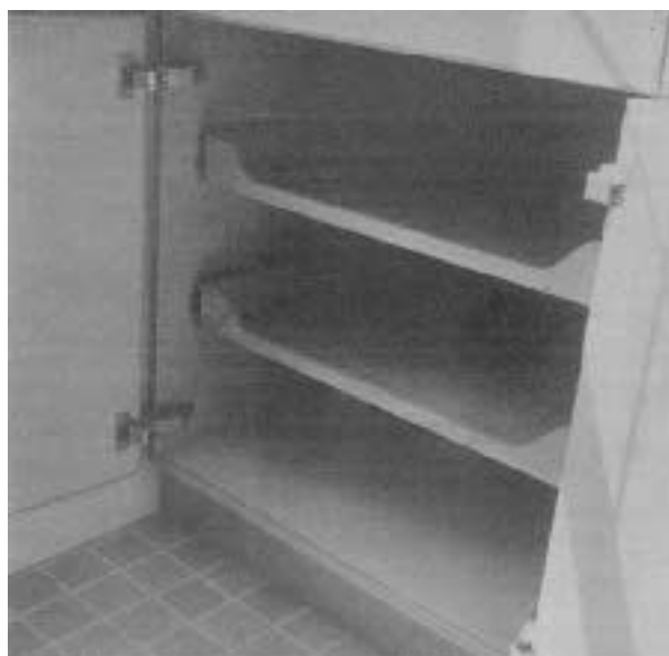
Figure 3. Although the Grass #1203 hinge opens only 170 degrees, it swings the door out of the way, so it will not obstruct drawers or pull-out shelves.
