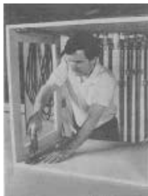
Figure 9. Place the case on its side to install the slides. It's much easier to work with gravity than against it.
