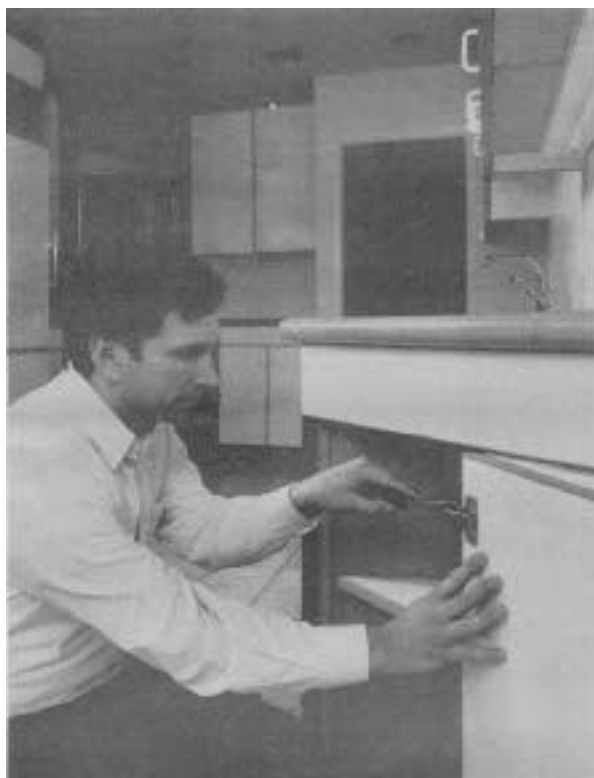
Author Paul Levine makes final adjustments on the cup hinge of one of his custom cabinets
