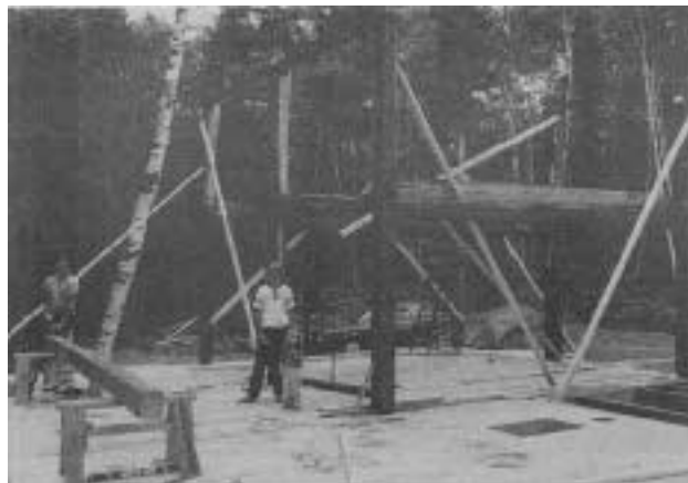
Safe assembly requires a good working knowledge of the original framing sequence and the soundness of the timbers. In this case, it was important to raise the earliest (1680) portion of the frame first.
