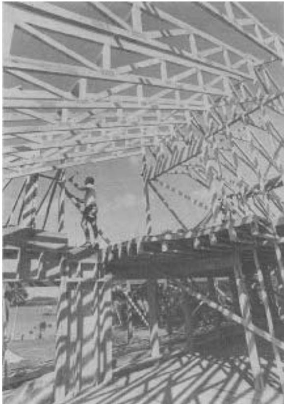
This is the first house in Florida built of fire-retardant-treated wood. It's Type-A rating from Underwriters Laboratories qualifies it for use in high-humidity environments.
