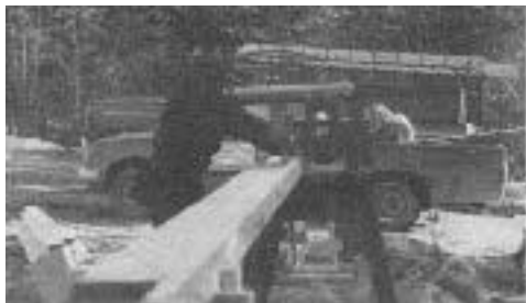
A radial-arm saw with two 12-foot extension tables is set up on every job (left). Using jigs and stops, the saw is used to pre-cut everything (right) with speed and accuracy. But temporary electrical service, says the author, can create big problems.
