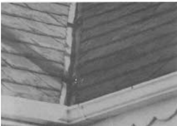
The cold-tar repairs to this valley will not last long. The flashing is copper and is appropriately installed in stepped sections—but it still failed before the slate roofing.
