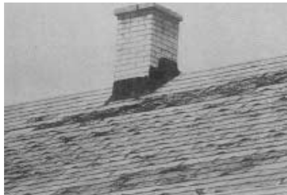
These shingles have buckled into "birds' mouths," caused by aging and a lack of attic ventilation.
