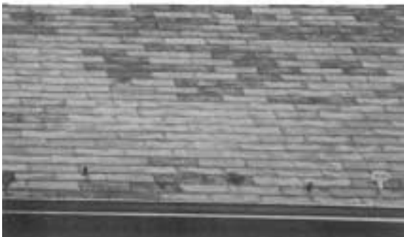
Not all slate is created equal. White efflorescence and brown stains indicate that these 40-year-old slates are delaminating and absorbing water, and have only ten or so years left of useful life.
