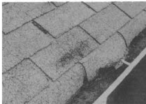
These drooping shingles lack support from either a wood or metal starter course. A properly installed metal drip edge will support the first course and direct rain into the gutter.
