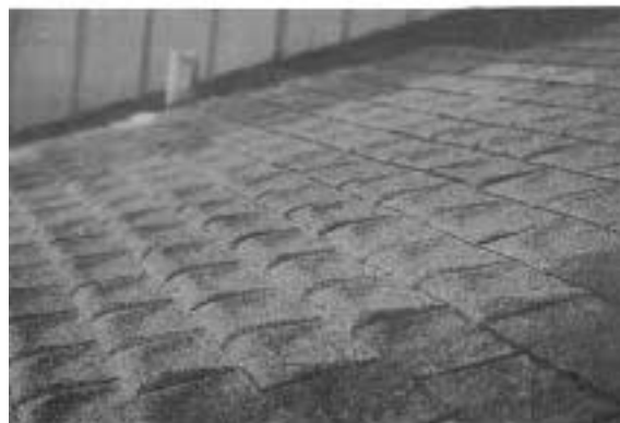
In the 1970s, some manufacturers skimped on the amount of asphalt coating on the underside of the shingles—causing them to cup.
