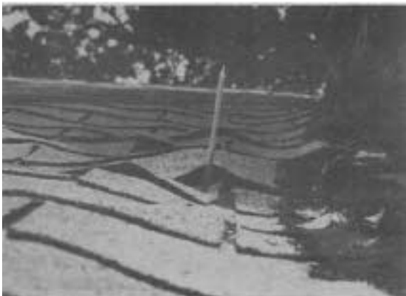
Older chimneys were flashed through to the flue tile. Few modern chimneys, however, are flashed correctly. Common mistakes are no base flashing, no counter-flashing, or too shallow penetration into the masonry. Leakage around this chimney led to rotted plywood decking.
