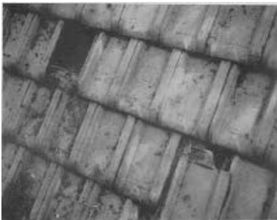
Clay tiles, like slate, are vulnerable to physical damage. Since clay tile is not waterproof, the membrane beneath the tile must also be inspected for leakage.
