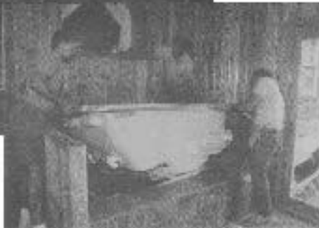
A pre-packaged spa goes in one, two, three, assuming the surround is level and correctly dimensioned. In this installation, access to the motor is from the basement stairs, just to the left and below the tub.
