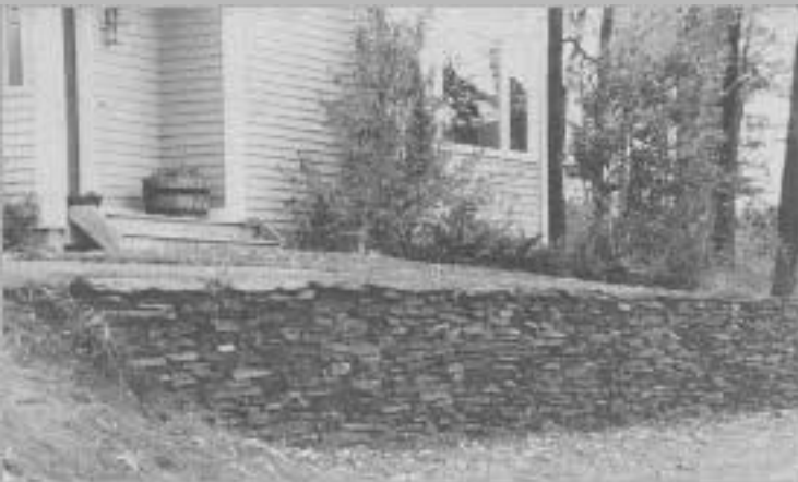
Dry stone walls (top) should be wide at the bottom and have a slope or "better" into the hillside. The taller stone structure (bottom) is actually a type of crib wall called a gabion. Gabions are made by stacking stone-filled wire baskets. They offer good drainage and can tolerate frost heave.
