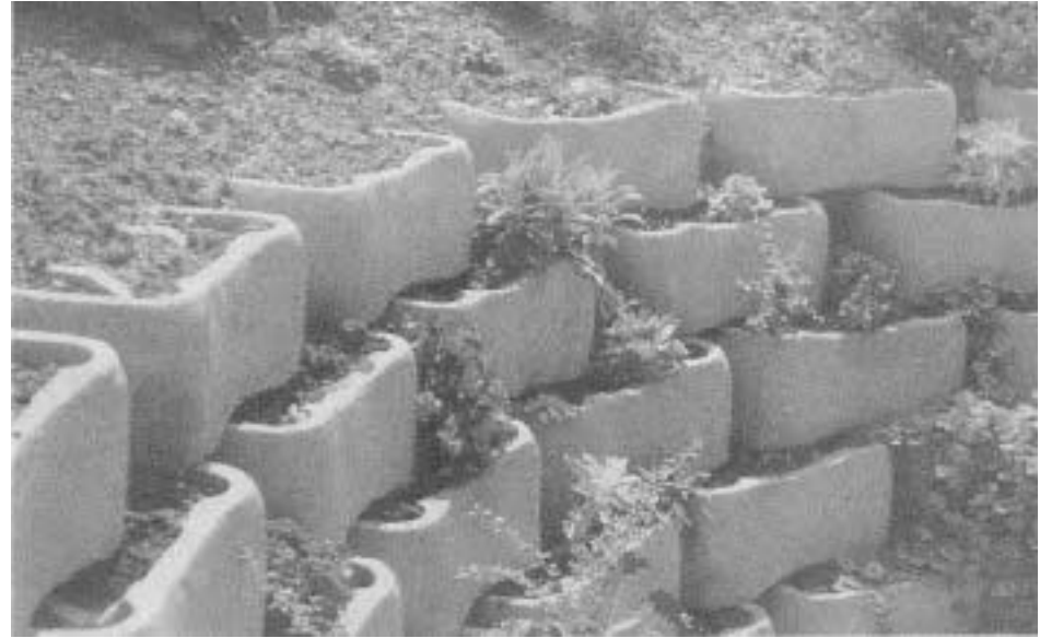
Precast Loffelstein blocks are set in a staggered arrangement to form a low retaining wall. The blocks—designed to support plantings—are available from Silidur North American Co., Illyria, Ohio
