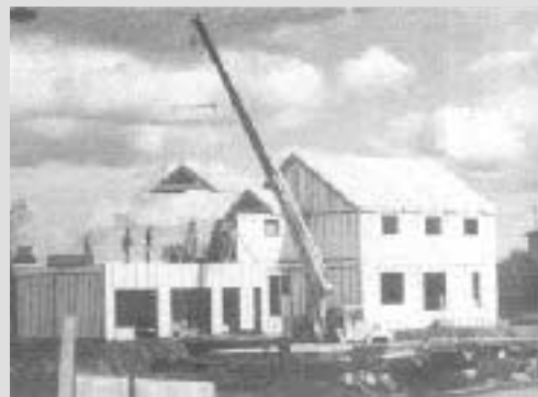
Three to four days of crane time are needed to assemble the shell. Notice exterior strapping is used to maintain an air space between wood siding and foam sheathing.
