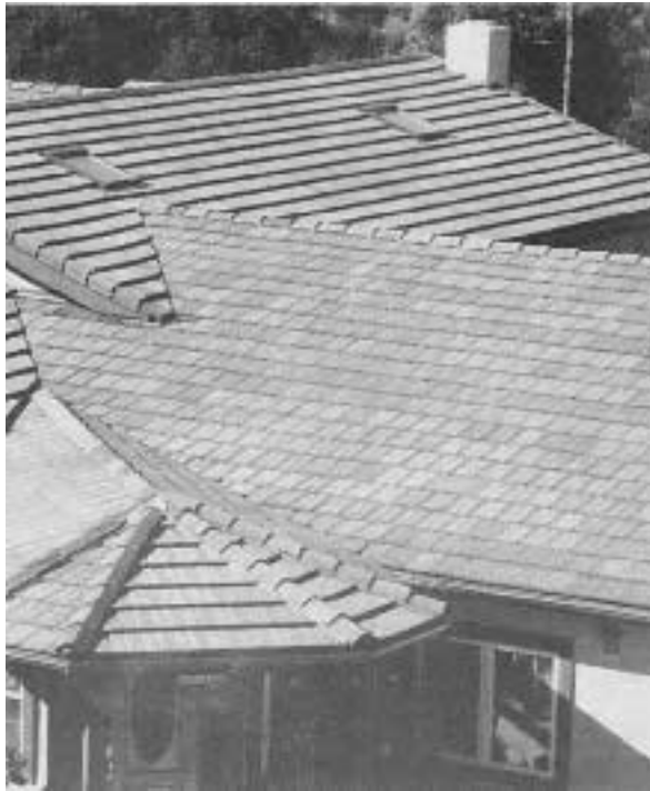
Concrete Tiles. One major difference between these "shakes" and the real thing is their fire rating. Shakette concrete-roofing tiles are completely incombustible.
