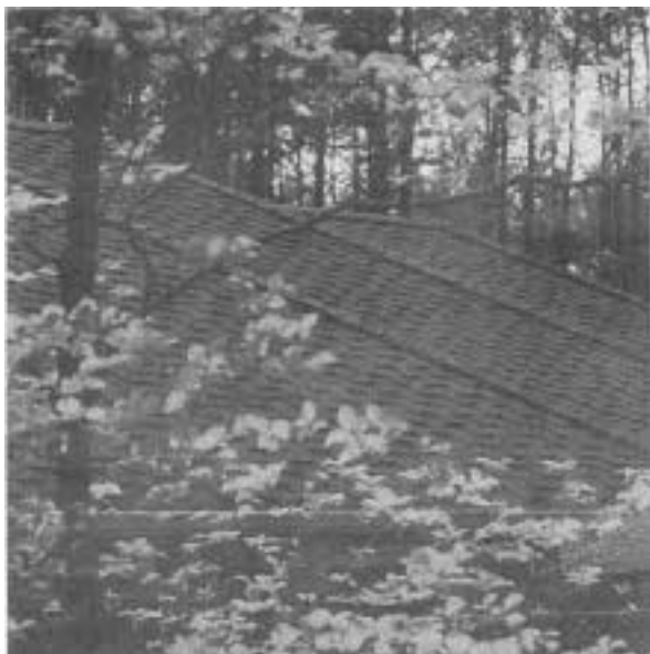
Wood Shingles. These wood look-alikes are actually made from asphalt. Extra weight and curvature of the edge gives Celotex's Presidential Shake its dimensional look.
