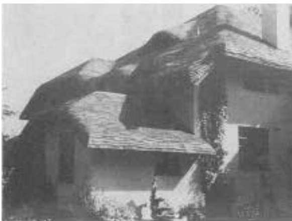
Bent Cedar. Even though this roofing may seem intimidating, Country Cottage Roofs maintains that it's easy to install. They sell specially-designed framing components that enable builders to frame the roof with conventional procedures and attach their component system to the existing framework.
