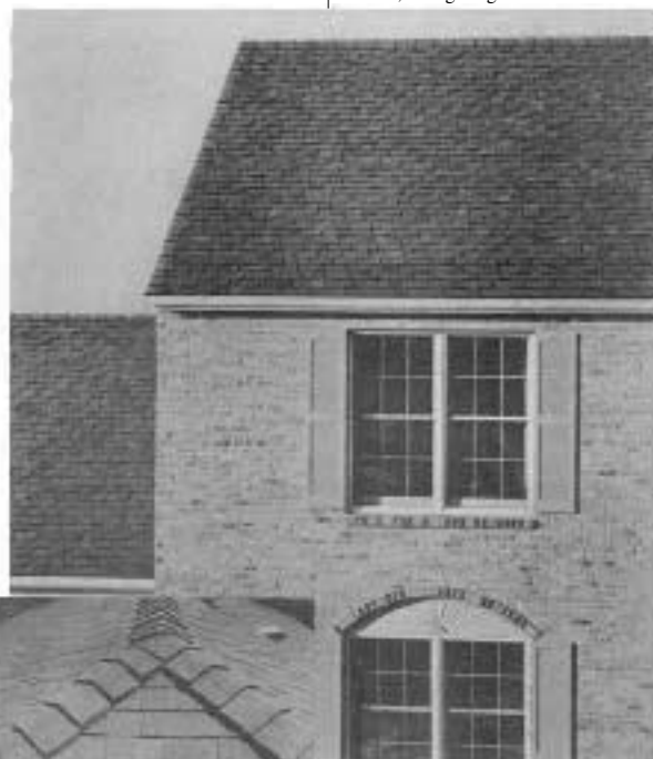
Wood Shingles. This roof features the Summit Shingle, Georgia Pacific's approach to the "wood shingle" look. The shingle has a 5 1/2-inch exposure, making them very close to wood shake size.
