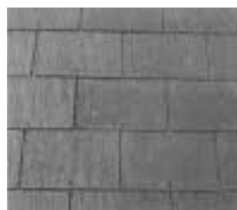
Cement Shingle. Eternit makes this roofing "slate" out of fiber-reinforced cement.
