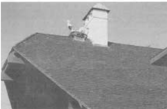
Luxury tiles. The tile on this roof may look hundreds of years old—but actually they were recently blended on site in hues of smokey reds and blacks to give a historic look to the building. The tile, called Norman, is one of Ludowici-Celadon's top-of-the-line shingles.
