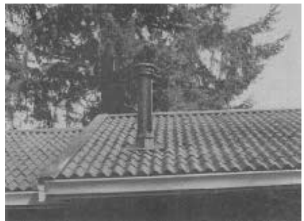
Asphalt sheets. Onduline's asphalt-impregnated roofing is promoted as an alternative to galvanized steel, but has the look of a tile roof. It's said to be impervious to acid rain damage.
