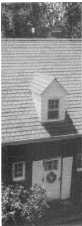
Slate Shingle. Slateline is one of the new architectural shingles out from GAF.
