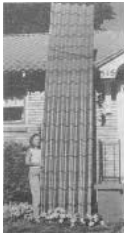
Steel Tiles. Because of their light weight, Met-tile steel panels (left) can run as long as 16 feet and still be manageable. (Steel weighs one pound per square foot, as compared to clay or concrete's 7 to 10 pounds.) The "clay" look-alikes on the residential complex in Houston (right) are Stile-brand steel panels and also come in lengths up to 16 feet.
