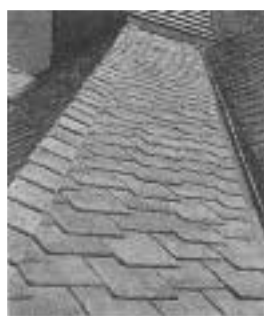
Mineral Fiber Slates. This roofing looks like slate, but is actually made from mineral fiber. Architectural effects can be achieved by blending a combination of colors or by simply staggering the butts.
