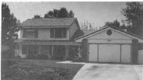
Lightweight Concrete. This roof did not require any special reinforcement. Made from portland cement, silica, and cellulose fiber, MaxiTile has less than half the weight of clay or concrete tile.
