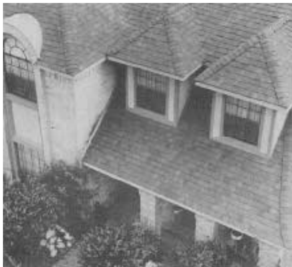
Wood Shingles. This house is roofed with Oakridge shingles—Owens Corning's version of the fiberglass "wood shingle."
